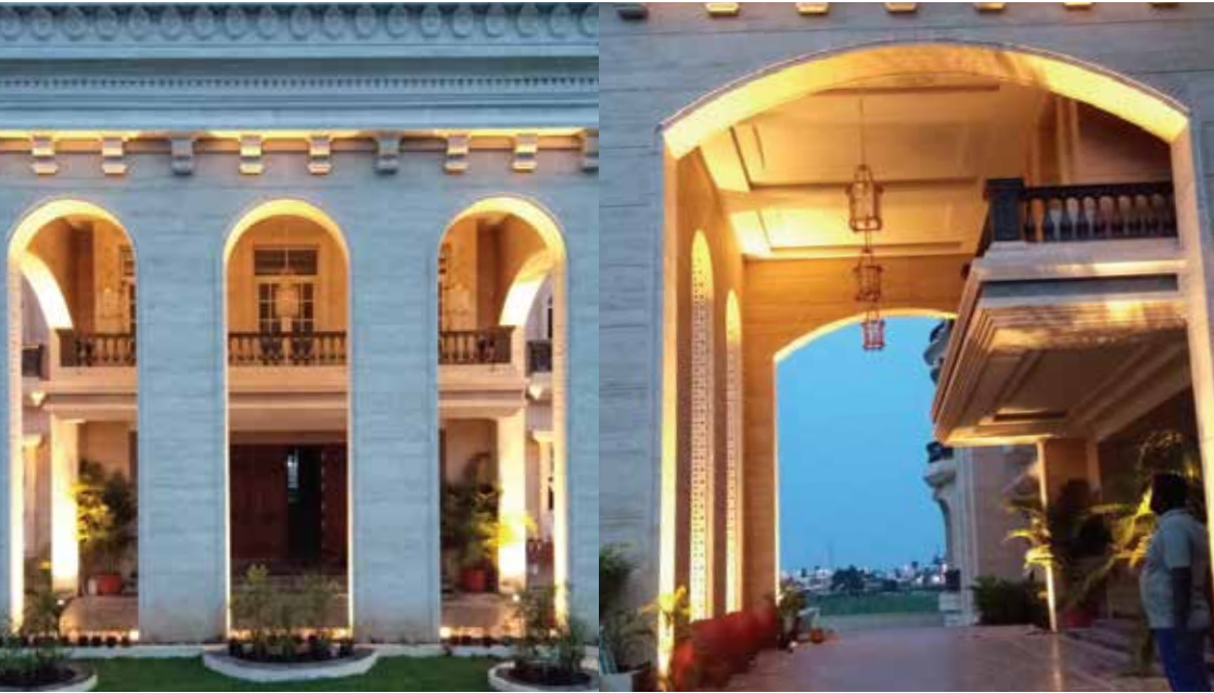
PRIVATE RESIDENCE, CHENNAI
